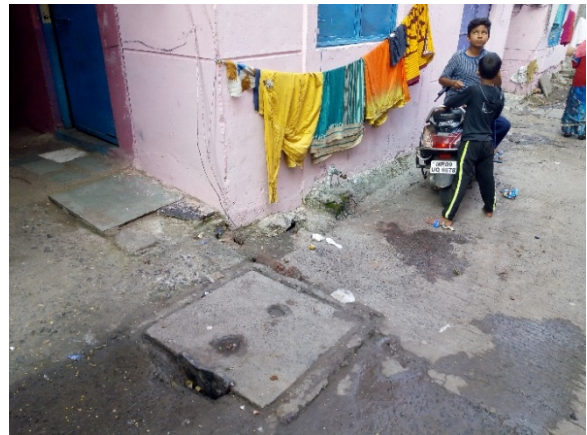
Inspection chambers often overflow. Photo: CURE, 2019.
