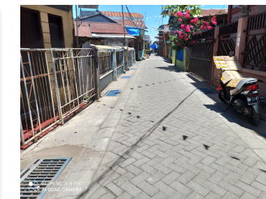
In 2020 Kotaku completed work to prevent flooding, including a concrete fence (left), closed drainage, and a better road (right).
