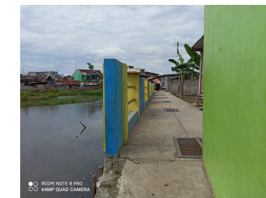
In 2020 Kotaku completed work to prevent flooding, including a concrete fence (left), closed drainage, and a better road (right).
