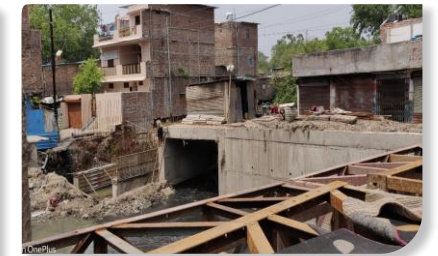
One arm of the permanent concrete bridge is complete (left). The second arm is still under construction (top).
