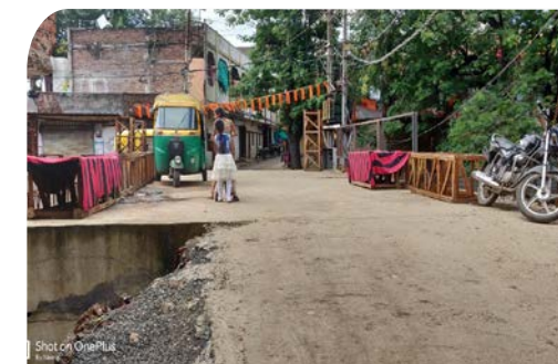
One arm of the permanent concrete bridge (left). Safety railings were added to both arms of the bridge (right).
